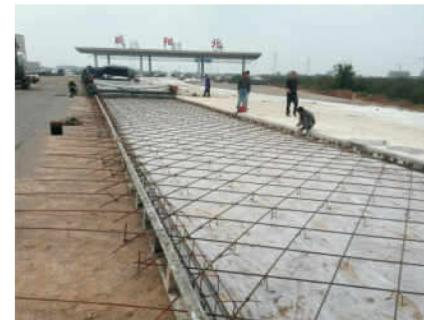
预应力钢筋 Prestressed reinforcement
